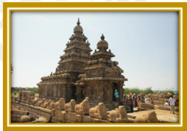
Figure 7: Architectural features of the temple, one of a series of sea-coast temples built in Dravidian Architectural Style under the patronage of the Pallava kings in the 7th and 8th centuries.
